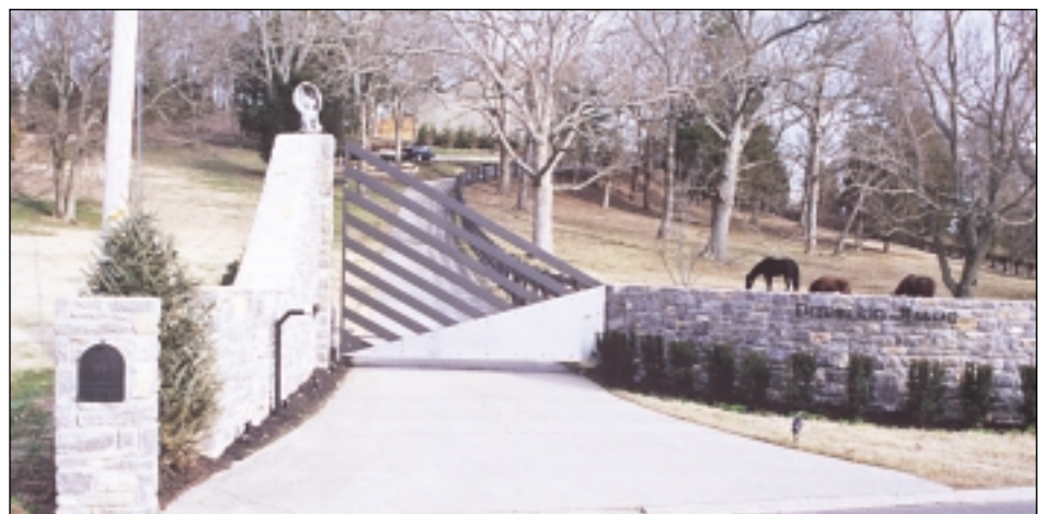
Herndon & Merry teamed with architect Thom Meek to produce this unusual entrance gate of wrought iron and stainless steel
