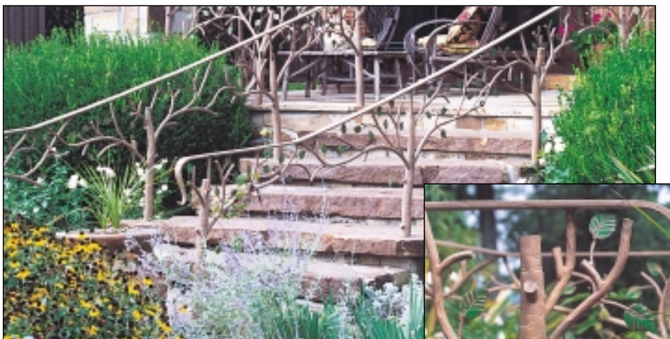
One of the most unusual designs ever executed by Herndon & Merry is the "tree railing" commissioned by Steve and Terri Smith; the close-up shows the realistic trunk, branches and leaves, all made of iron.
